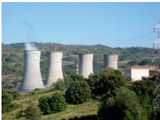
Geothermal cooling towers at Larderello, Tuscany (Italy) Photo: Simon
