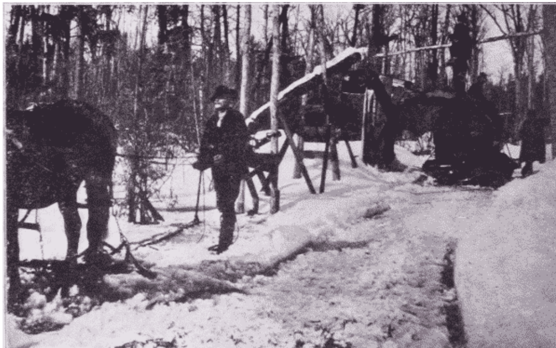
Fig. 10. Making an Ice Road by Flooding.
