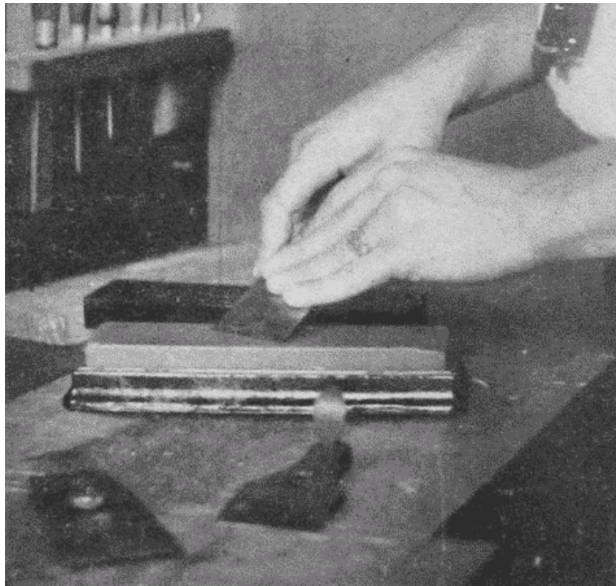
Fig. 77 Whetting a Plane-Bit.
