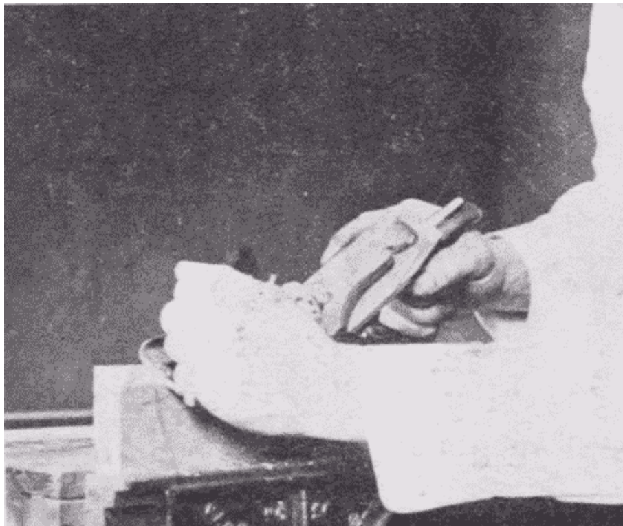
Fig. 272. Thru Chamfering.
