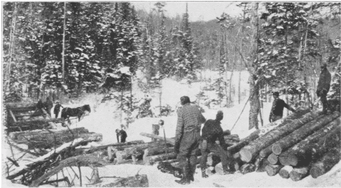
Fig. 12. Loading a Sled from a Skidway.
