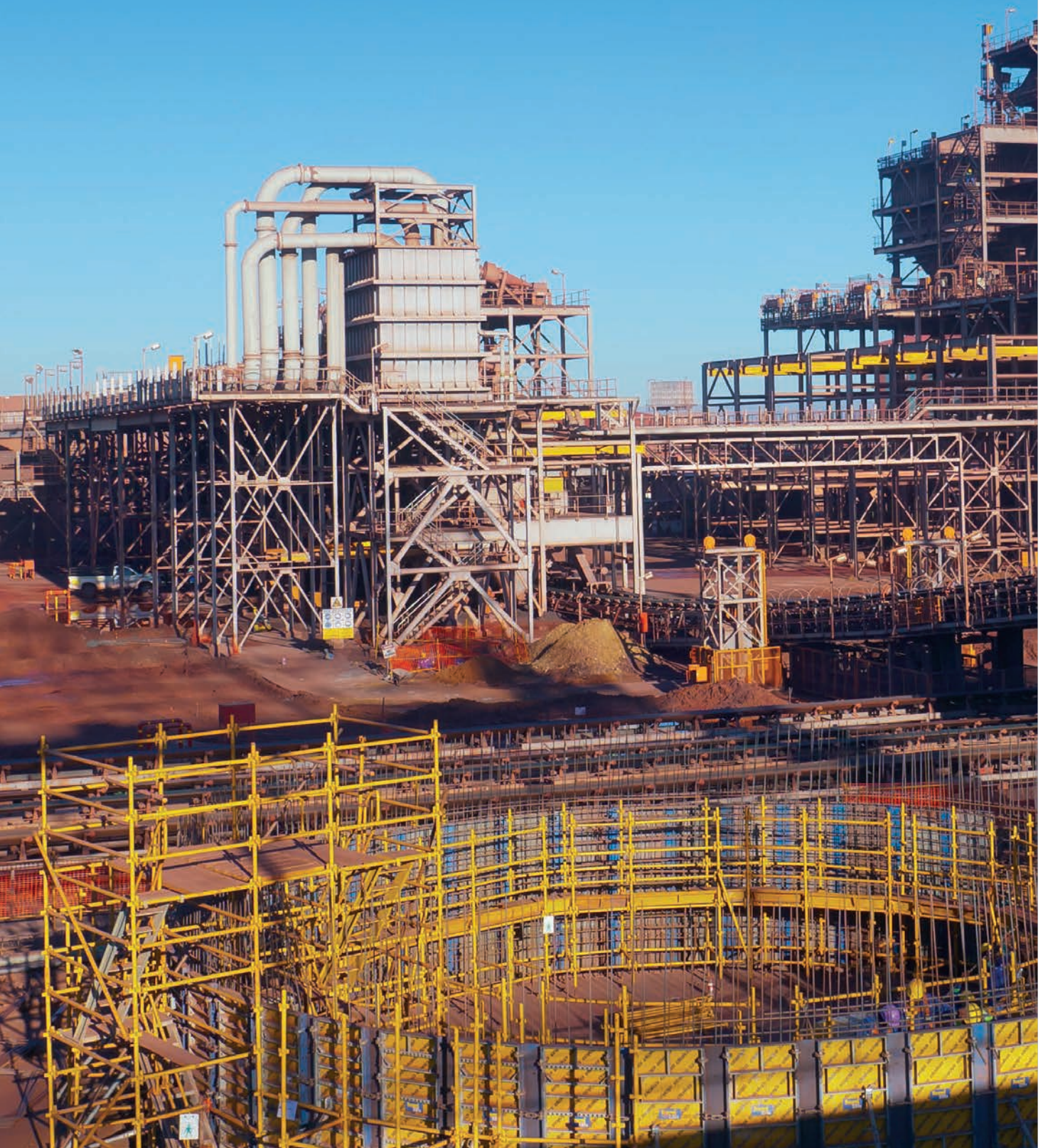
WHIMS plant under construction at Khumani Iron Ore Mine
