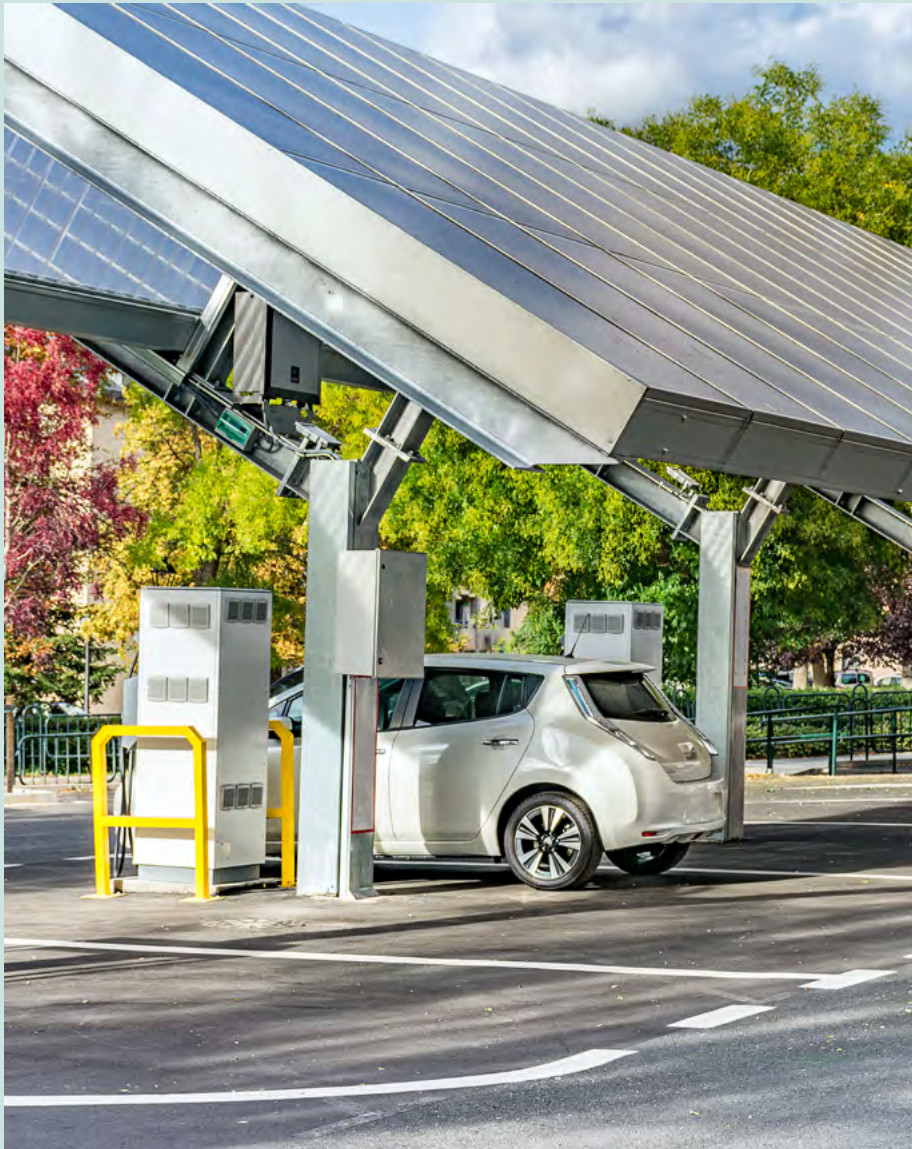
Spain: Car charging station for self-sufficient and first free photovoltaic panels in Europe.
