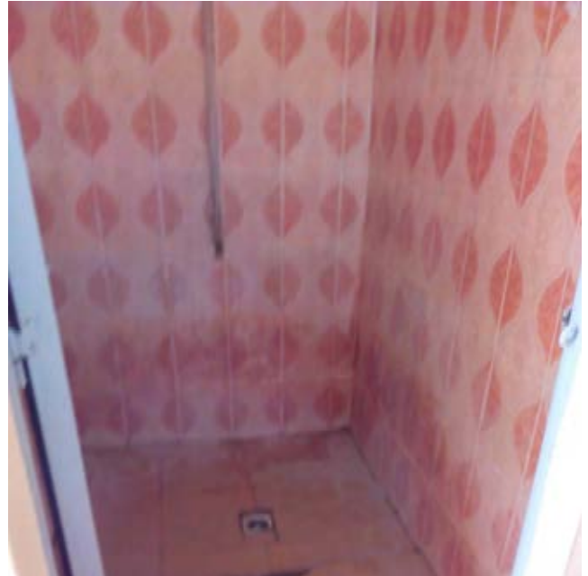
Photo 2.2 Improved toilet; no flush, but wet
