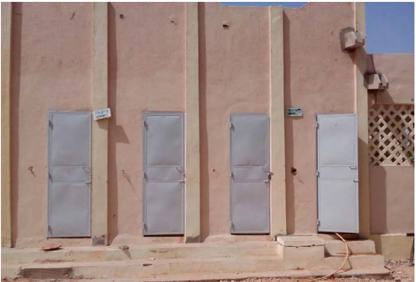
Photo 2.3 Improved pit latrine block
