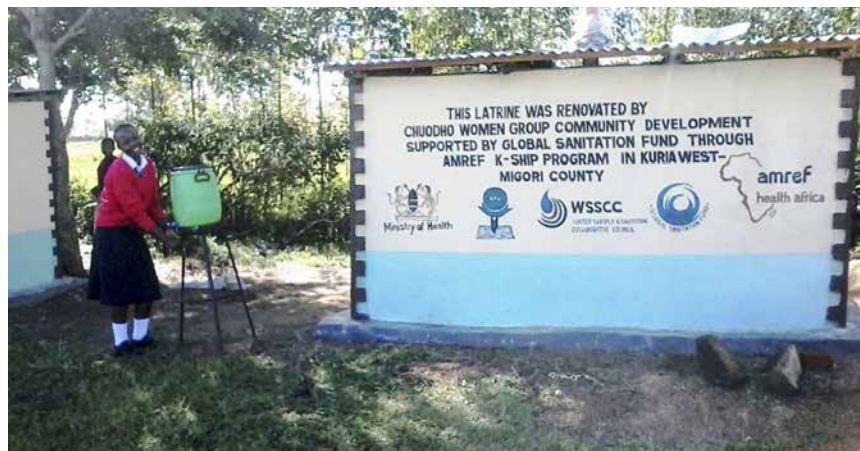
RENOVATED SANITATION FACILITIES AT NGISIRU PRIMARY SCHOOL. ©KSHIP
