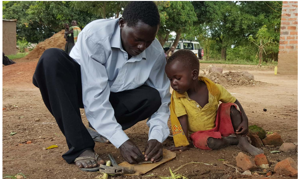
A MEMBER OF A GSF-SUPPORTED COMMUNITY IN UGANDA BUILDS A FLY-PROOF COVER FOR HIS LATRINE. ©WSSCC/USF
