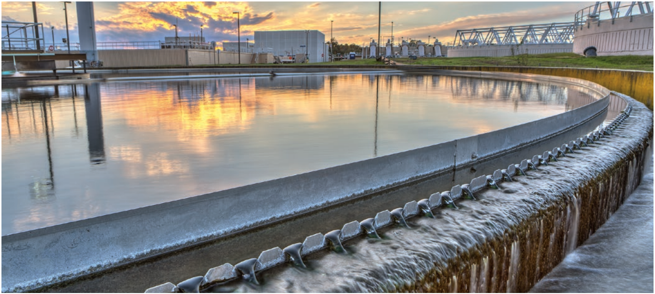
Water treatment plant in the U.S.
