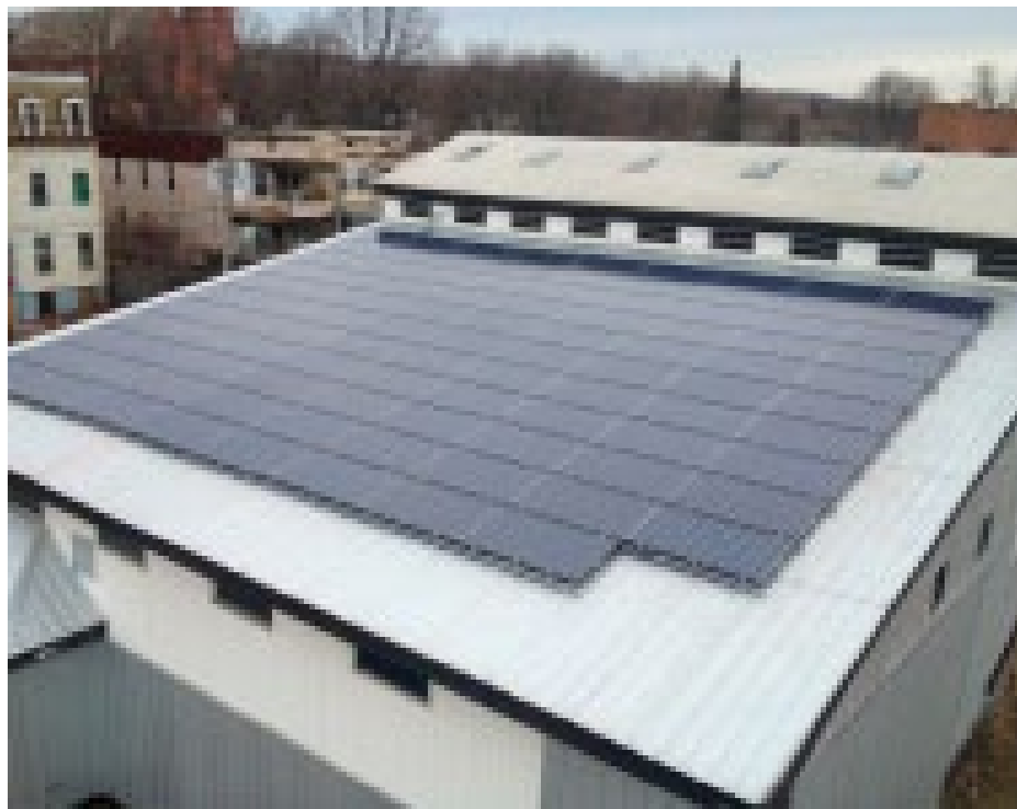
A commercial rooftop PV plant constructed by US Light Energy in Albany, New York.
