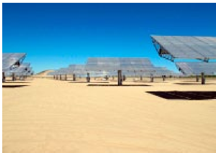
Soitec CPV modules in use. The South African Government Employee Pension Fund (GEPF) will become a long term investor in the 44MWp Touwsrivier solar CPV project.
