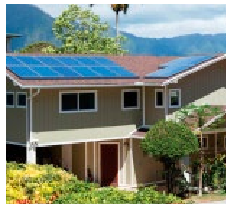
A SolarCity residential installation in Hawaii. SolarCity is offering US$70.2 million in 'Solar Asset Backed Notes' through its subsidiary, SolarCity LMC Series II.
