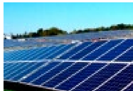
Strata solar Project, north Carolina. The company received US$100 million from Wells Fargo to invest in nine projects in the state.
