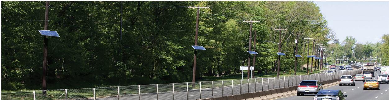
Figure 3-2: Petra Solar SunWave™ Installation in New Jersey on Utility Distribution Poles
