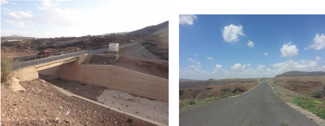
Figure 43. & 44. Road body used as recharge dam in asphalt road
