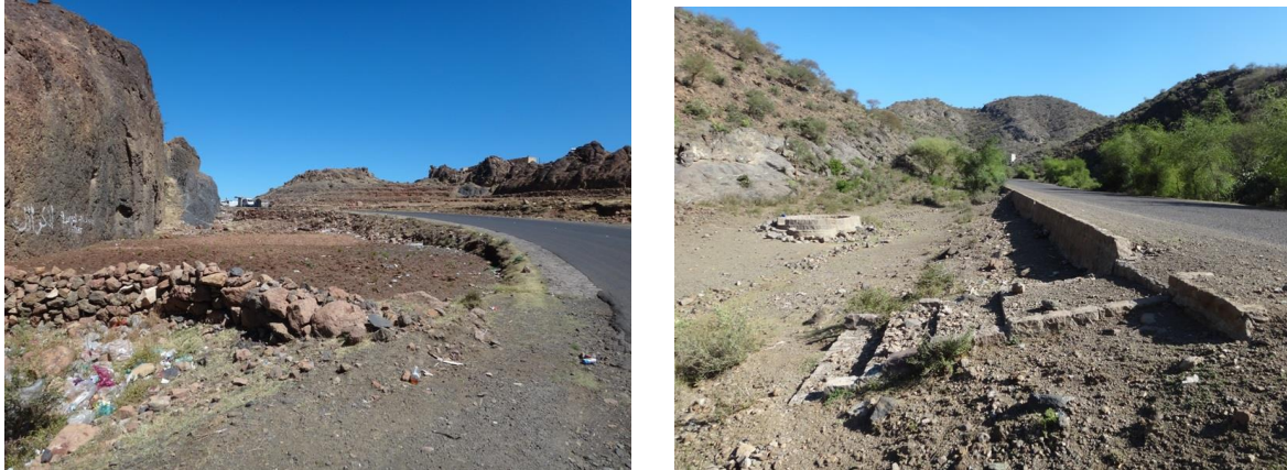
Figure 13. & 14. Flood water guider from roads (left) and stepped intake (right)
