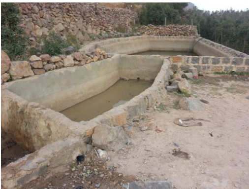
Figure 4 & 5. Ponds harvesting water from side drains
