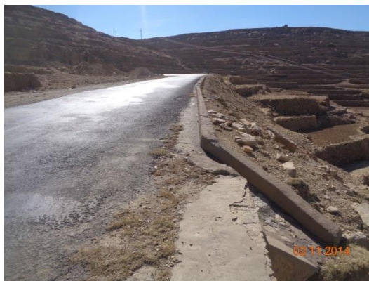
Figure 30. & 31. Erosion from uncontrolled run-off (left) and controlled road run-off (right)
