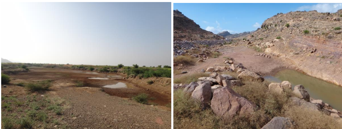
Figure 15. & 16: Farmers in Wadi Tabab AlKhabt - Mahweet district (Yemen) using a borrow pit in wadi Tabab near the road from Qanawis to Al-Mahweet as retention and recharge pond (left) Borrow pit cum recharge ponds near I-Rojom (right)
