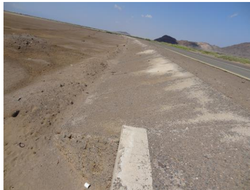
Figure 39. & 40. The embankment was protected by concrete and there is a small temporary bund to retain the water in the upstream (the potential is using gates in the culverts inlets).
