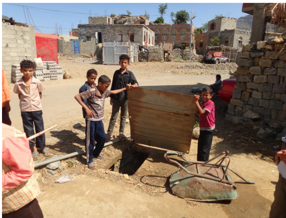
Figure 1. Water cistern filled by run-off from road-surface
