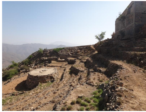
Figure 8 & 9 Cistern filled from road recharge and stone blocking first flush, Al Wastah
