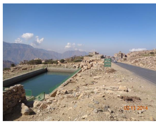
Figure 6 & 7. Road-run-off collected respectively from (up-slope) side drain and from escape in down-slope side drain
