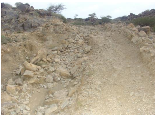
Figure 41. and 42 : Earthen roads risk developing into a flood path – proper design with rolling dips and spill overs required.
