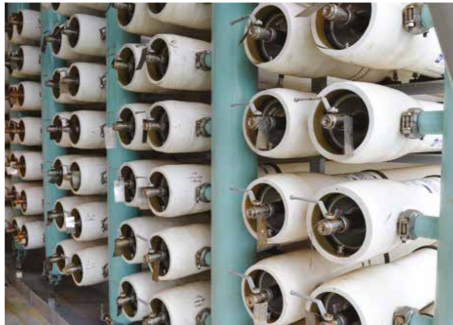
Caption: The water treatment system on PSVM.
