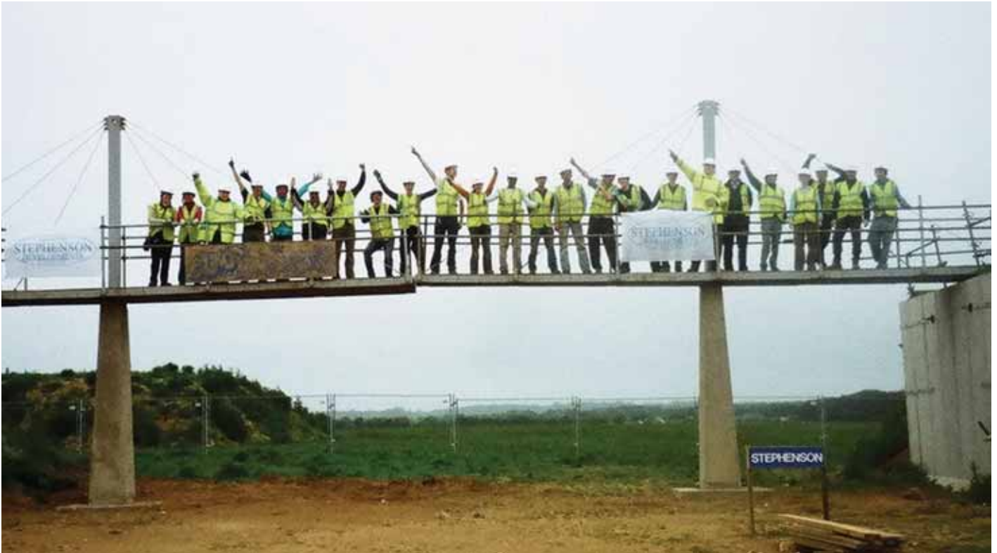
The final structure. Photograph courtesy of Jenny Auton
