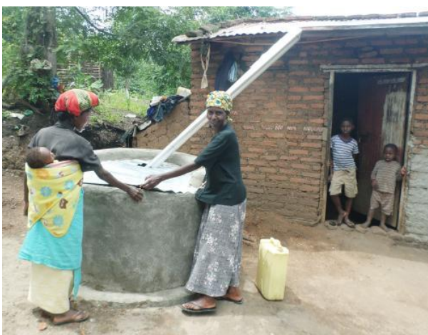
These water tanks can be self-made. Kighengi, Uganda. Photo: Kenja Thomas
